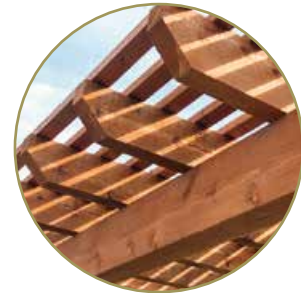
Braces Large 4x8 joists offer a beefy feel with the 2x3 purlins giving ample shade and comfort.
